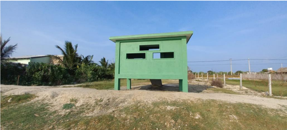
Figure 25: Bird Blind after the completion, January 2023
