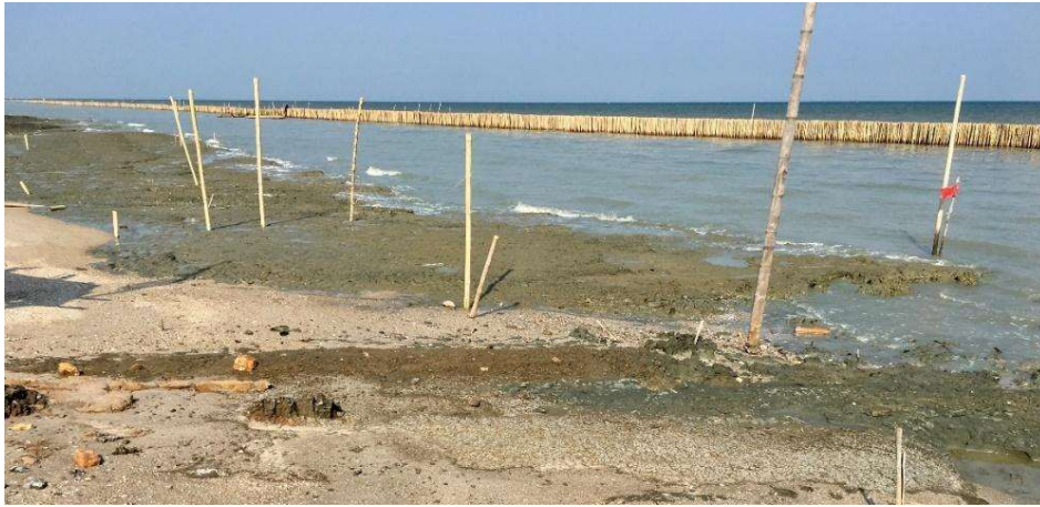
Figure 1. Bamboo fences erected along the shoreline for managing coastal erosion at Pak Thale.
